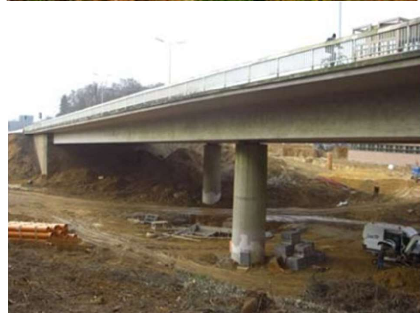
Views of the Champangshiehl bridge (Luxembourg)
