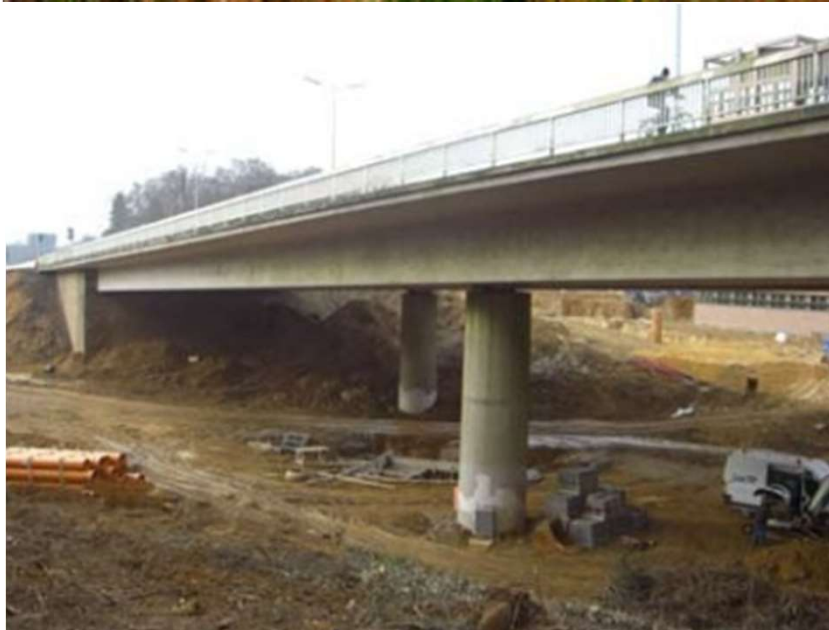
Views of the Champangshiehl bridge (Luxembourg)
