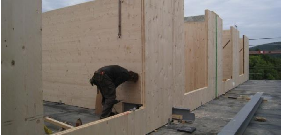
Figure 19: 2D plywood assembly early phase, Kierling, Austria © Architekturbüro Reinberg
