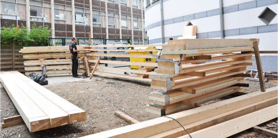
Figure 22: 1D timber elements assembly early phase, Brussels, Belgium © Atelier d'Architecture Galand
