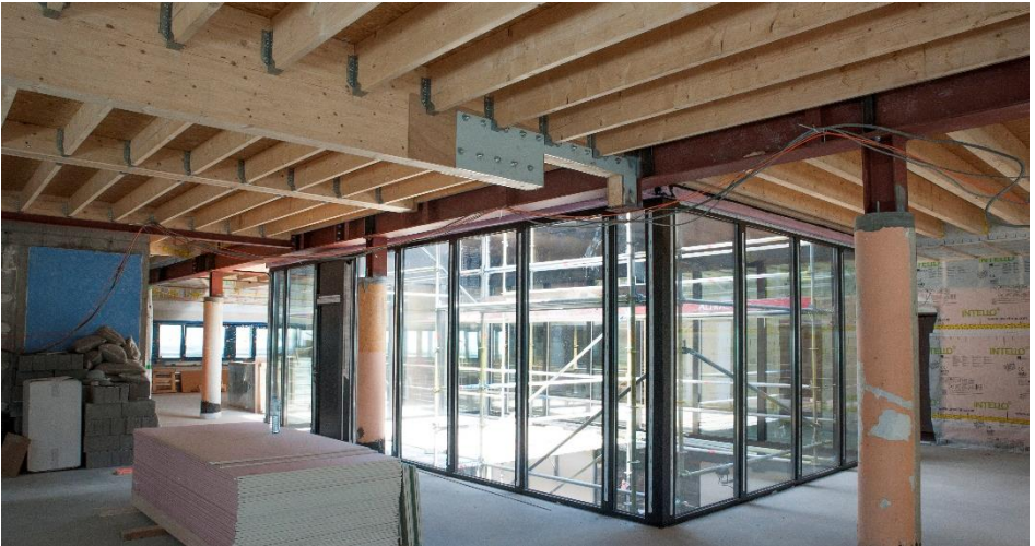
Figure 23: 1D timber elements assembly late phase, Brussels, Belgium © Atelier d'Architecture Galand
