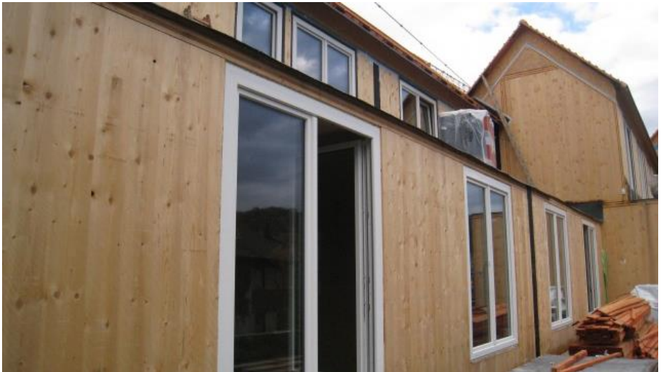
Figure 20: 2D plywood panels assembly late phase, Kierling, Austria © Architekturbüro Reinberg
