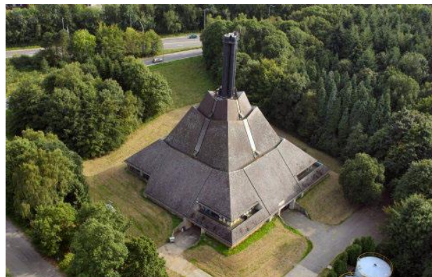
Figure 4: CHP plant of Sart-Tilman (Granulenergie, 2014)
