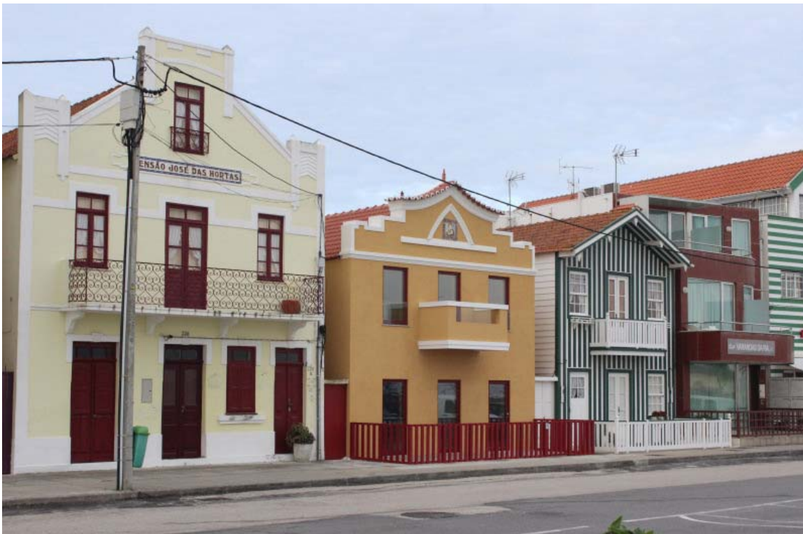
Figure 3.5.2: Passive House in Costa Nova, certified in 2016
