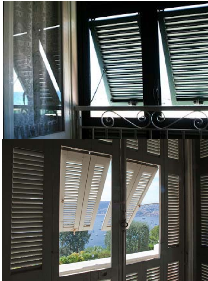
Figure 3.4.1: The Italian traditional “persiana” with the variant that allows lifting the lower part (“persiana genovese”)
