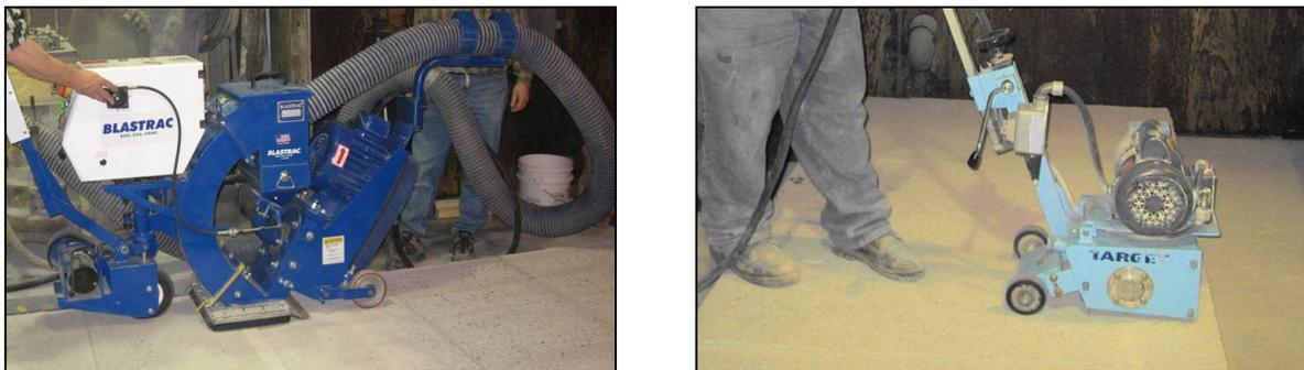
**Figure 3-5: Scarification and shotblasting surface preparation at CRIB (UL program)**
