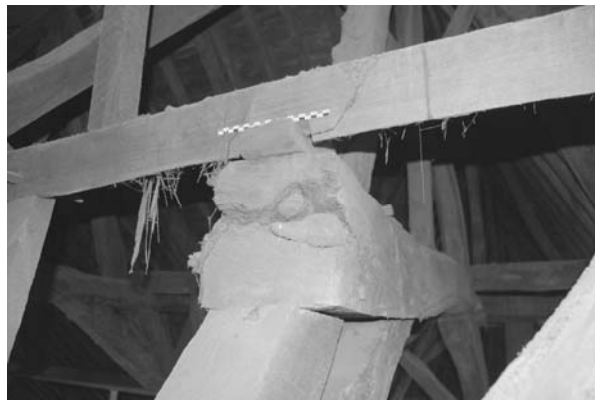
Figure 4 - Example of a fork in a tie beam near the assembly with the rafter. © SPRB
