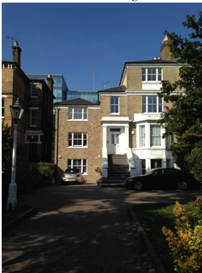
Fig. 20: Example of an extended and converted building
