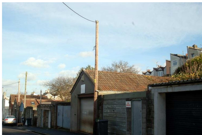
Fig. 42. Rear garages of Eldon Terrace
