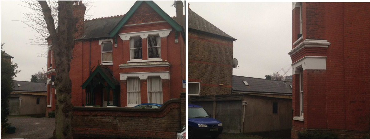
Fig. 11 & 12. Front of 14 Carlton Road, some signs of dilapidation (broken window)
