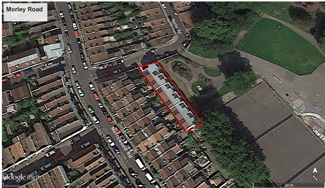
Fig 50. Aerial photo of Morley Road
