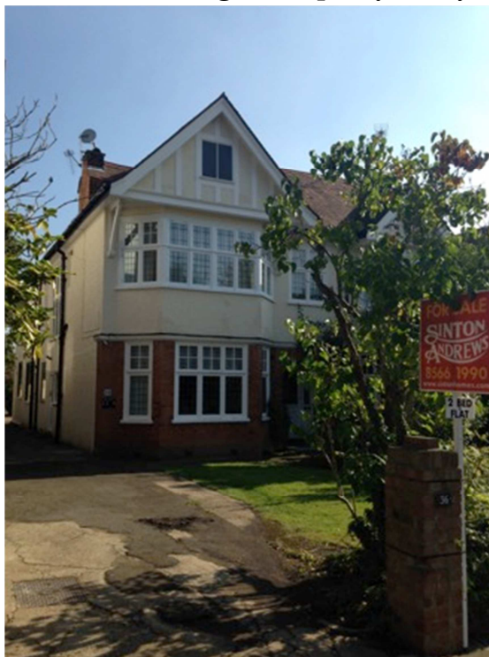
Fig. 21: An example of a conversion of a single occupancy family dwelling to four flats
