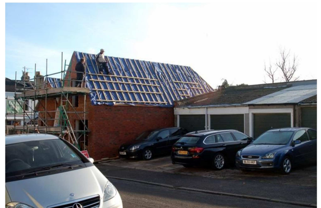
Fig 36. 1 Tyne Road, construction
