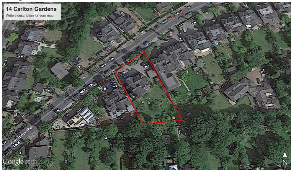
Fig 14. Aerial photo of 14 Carlton Gardens
