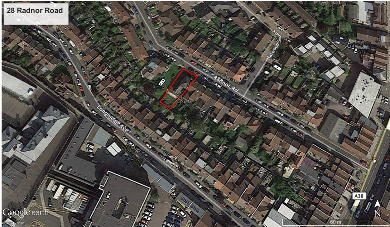
Fig. 31: Aerial photo of 28 Radnor Road
