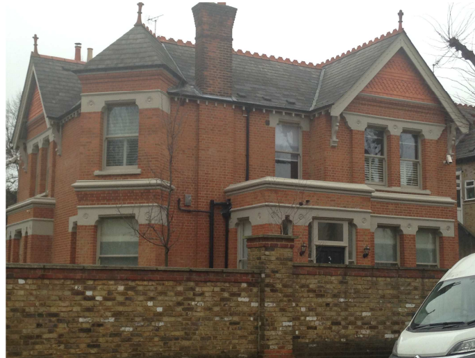
Fig. 13. Opposite 14 Carlton Gardens: recently redeveloped with security features
