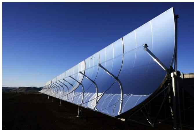
Fig. 1. Parabolic trough collectors (PTCs) connected in series (photo: SEGS III, California)
